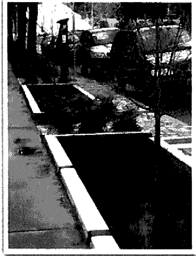
Roadside Rain Garden Example
